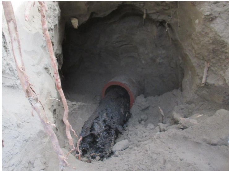
City Tree Roots Cause Main Sewage Line Back Up
