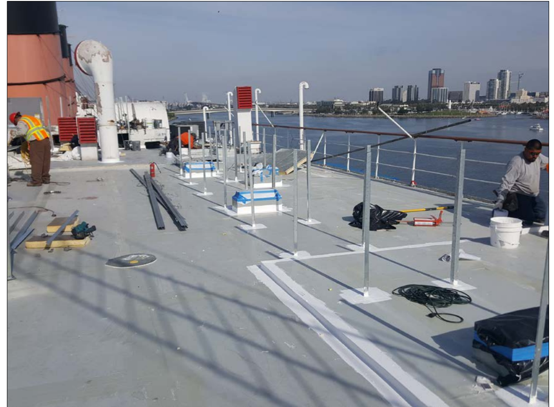
Roof damage and repair/waterproofing on Bridge deck (above Captain's Quarters)
