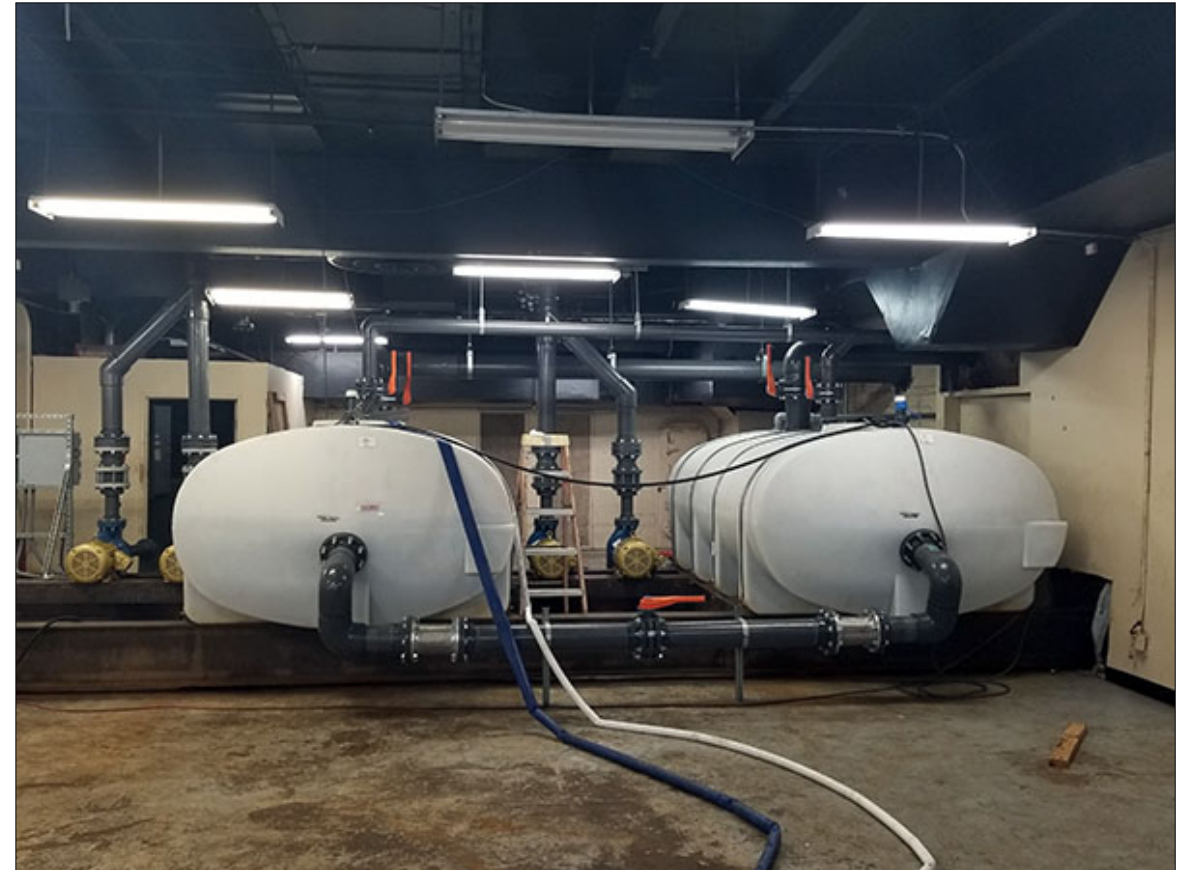
New temporary sewage tanks
