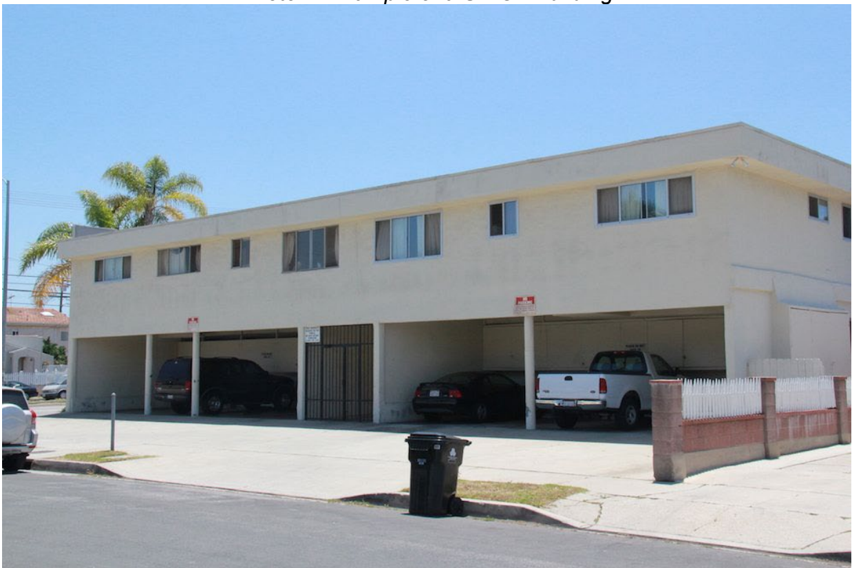
Photo 1: Example of a SWOF Building
