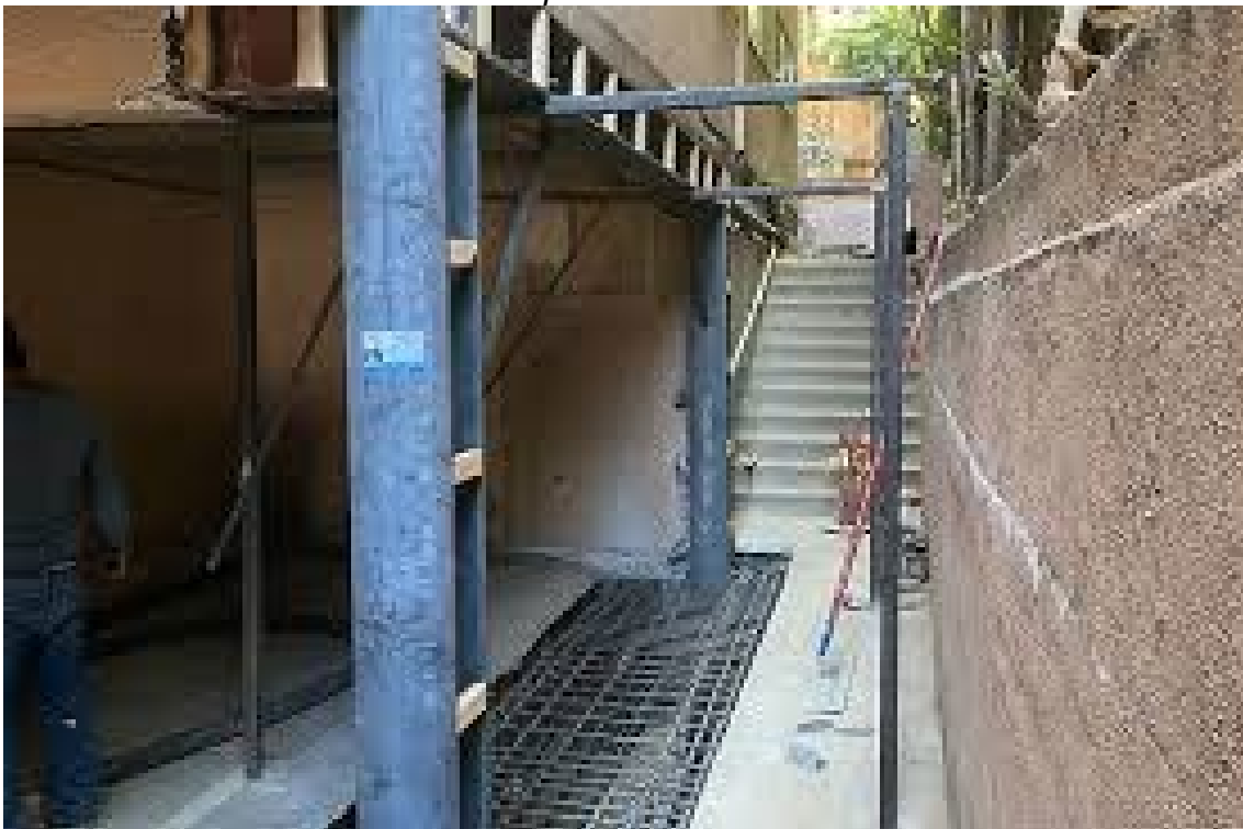
Photo 2: Example of a frame installation
