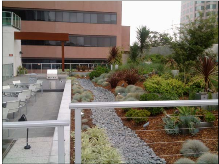
Bioretention (Planter Boxes)
