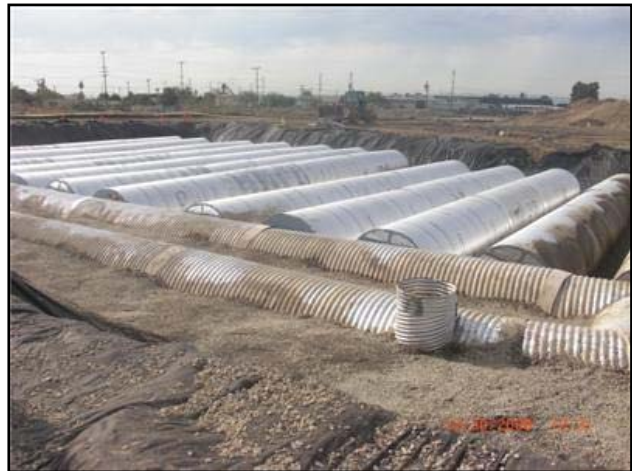
Underground Infiltration Units Lowe's, Pacoima
