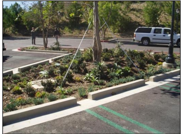
Bioretention in a Parking Lot Photo Credit: Geosyntec Consultants
