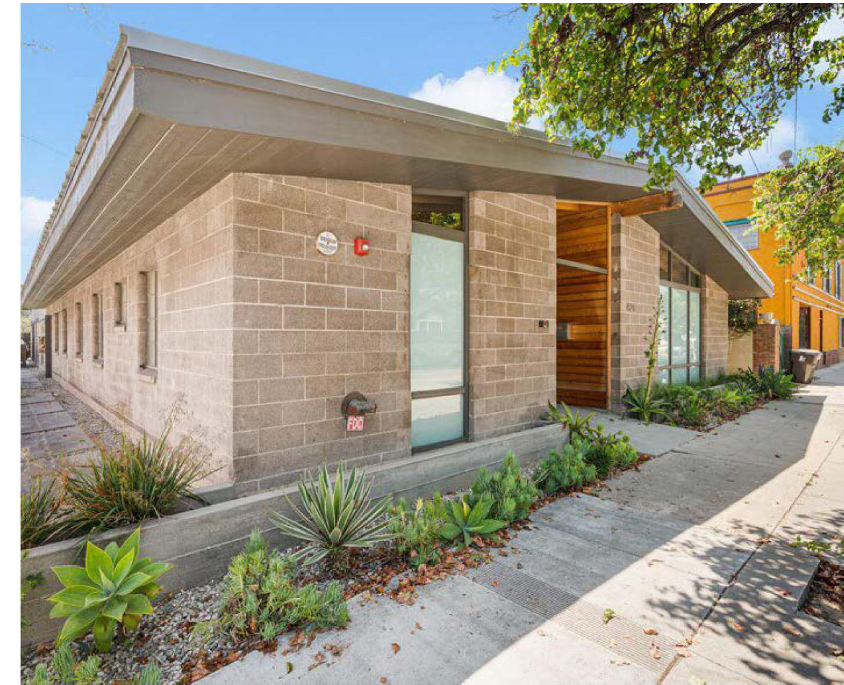
FRONT VIEW FROM NORTH
