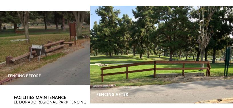
The Facility Maintenance staff replaced rotting rail fencing at the El Dorado Regional Park entrance culvert crossing at the entrance. The new fence is safer and provides great curb appeal improvement.
